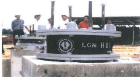
Installed SSI® on concrete foundation pedestal
