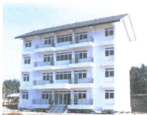
MRB / UNIDO Project in Indonesia 4-storey building in Pelabuhan Ratu, Java
